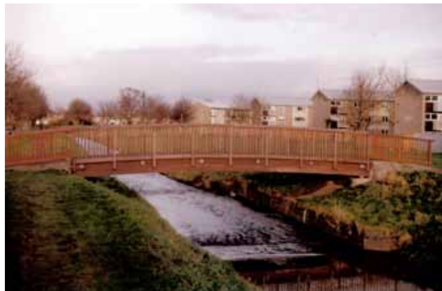
Dodson Macrae timber bridge, Grangemouth
