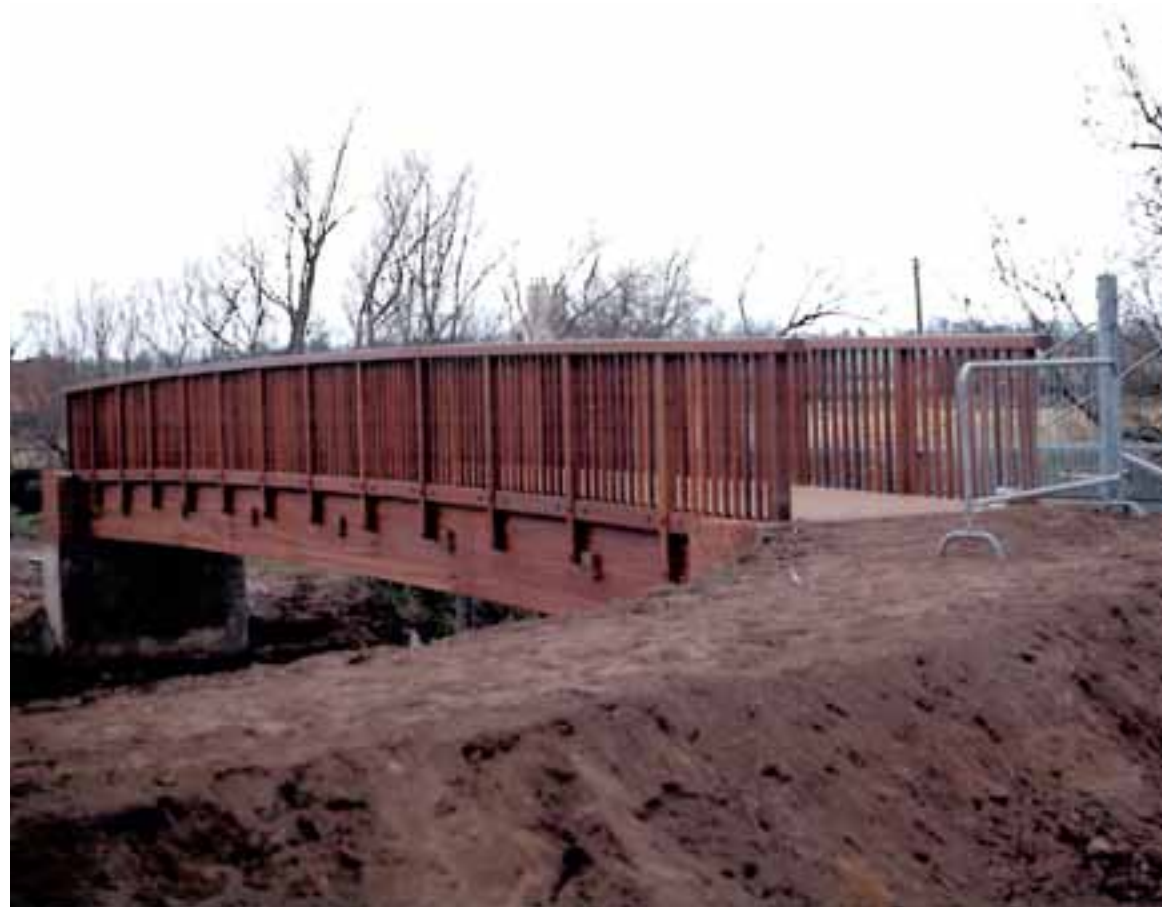
Dodson Macrae timber bridge, Knowes Farm, Dunbar
